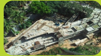
Construction in progress at the IME site (Top view)
